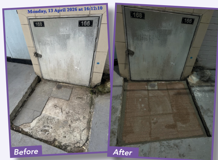
Repair of Flooring at Block 508 Jurong West Street 52
