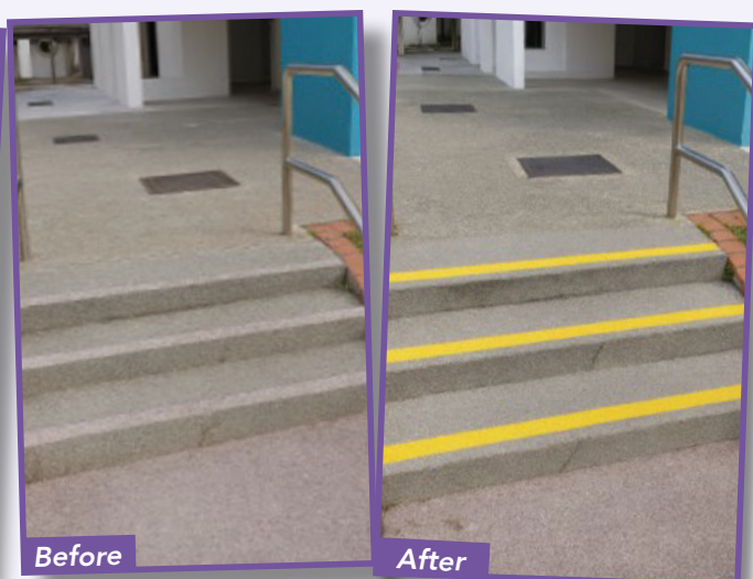
Step Edge Marking at Block 622 Jurong West Street 61
