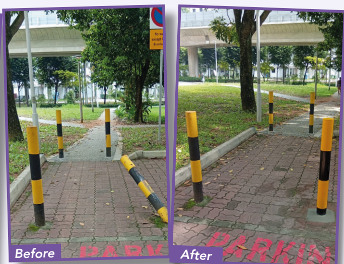
Replacement of Parking Bollards at Pioneer Zone 7
